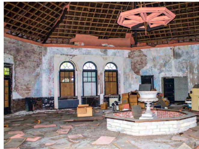
DAMAGE FROM MOISTURE INFILTRATION AT BUILDING #6
