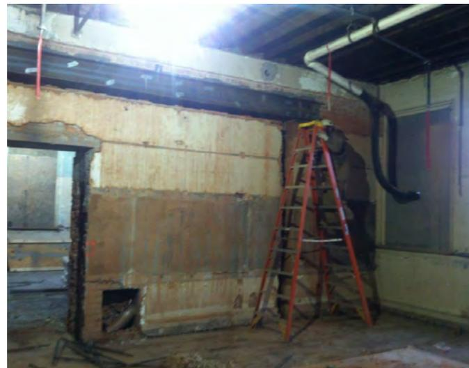
CONSTRUCTION PHOTO SHOWING REMOVAL OF BEARING WALL
